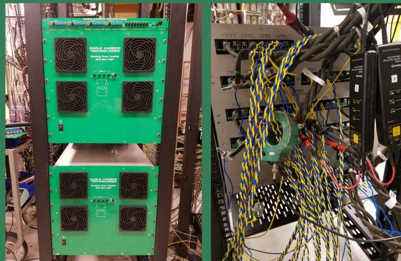
Left: Two of four SPAs delivered to HIT with the fiber-optic controller and interlock controller. Right: Back of SPA connected to HIT resonant circuit with current and voltage measurements shown.
